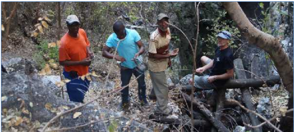
Figure 25. Two engineers from the Ministry of Agriculture, Water and Forestry (left) installing a water level data logger with the assistance of Willem Kubeb and Johan le Roux.
