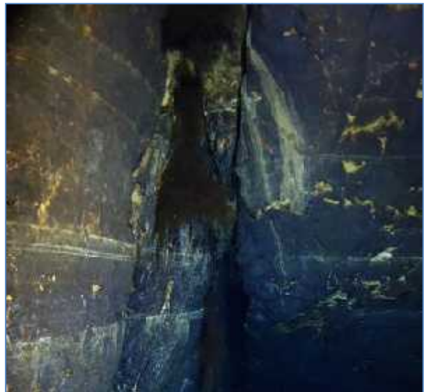
Figure 12. Calcite lines on the cavern walls below the May 2014 water level.
